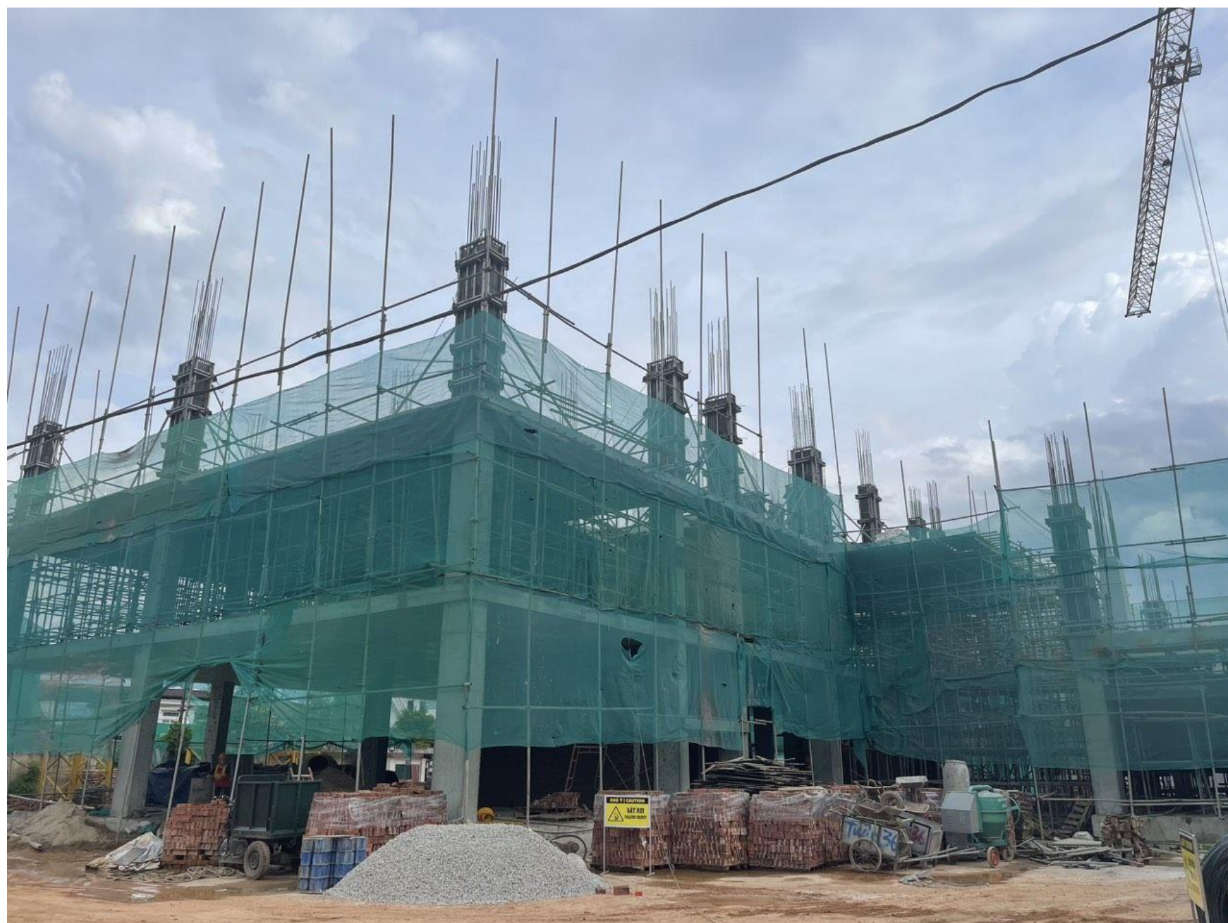
Construction images at Lang Son TNH Hospital
